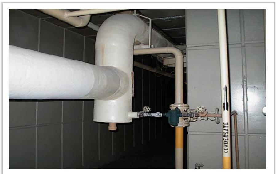
Figure 1 Steam Line Drip Pocket
